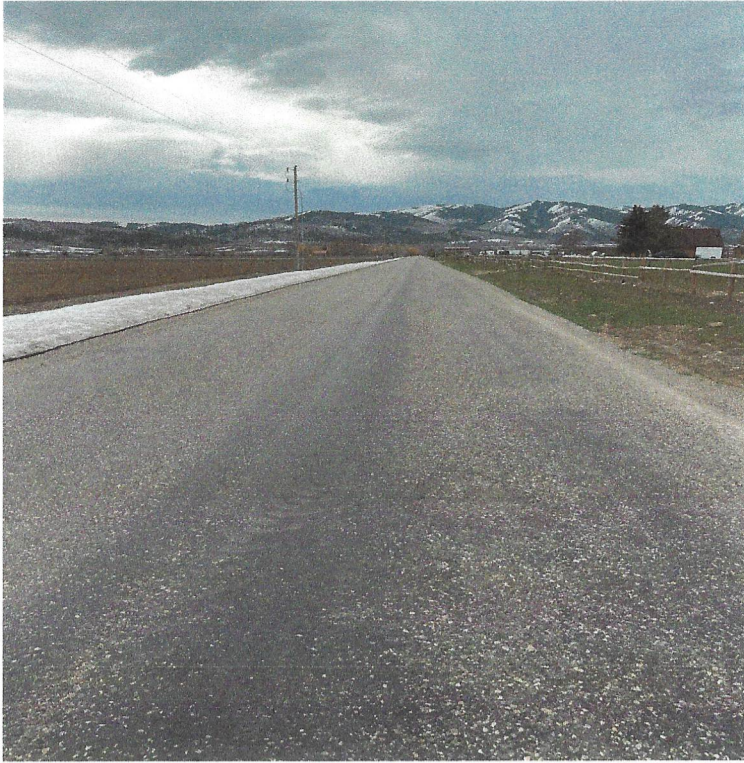
County Road "W9500S" which "Wisdom Way" will access. West view from intersection with "Wisdom Way"
