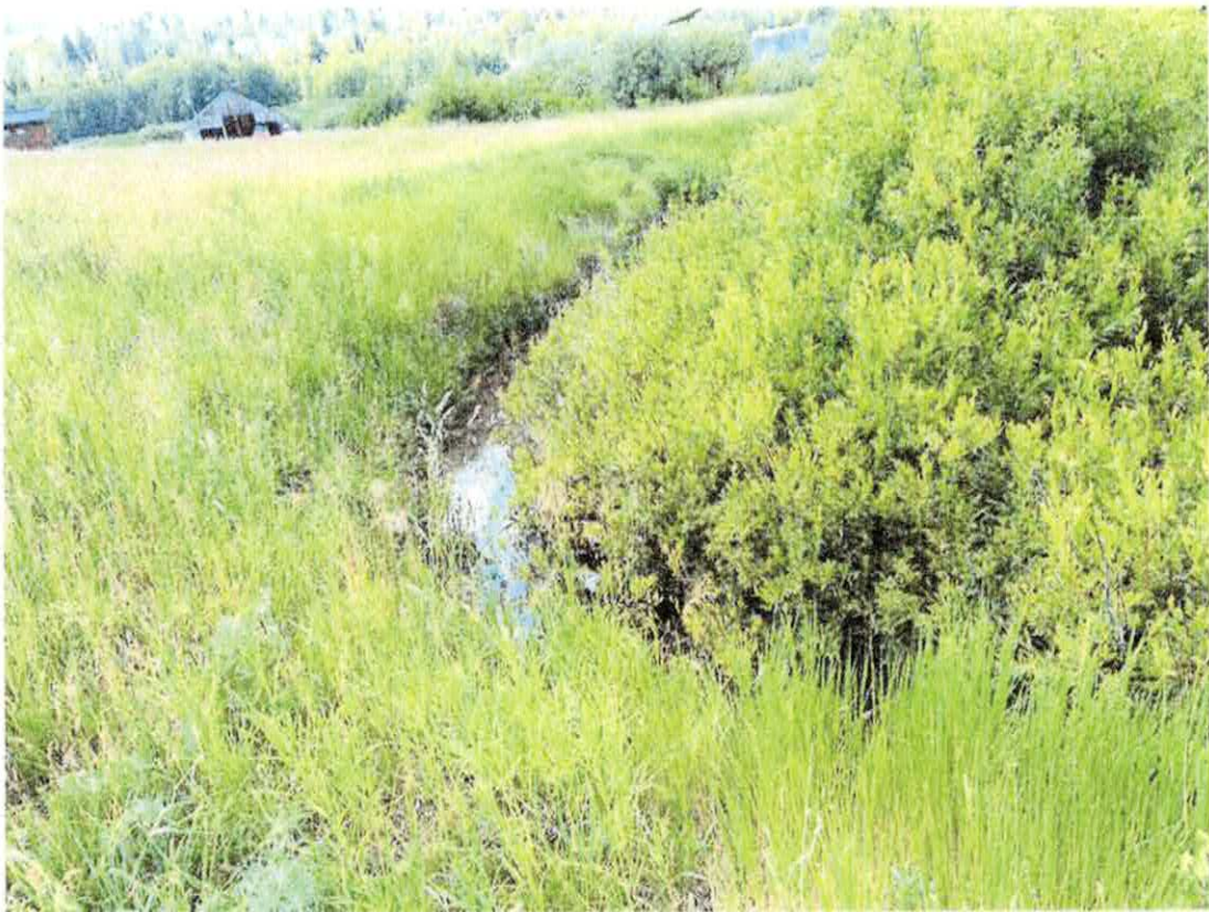
BOQUET CREEK INLET AREA NEW 24" CMP
