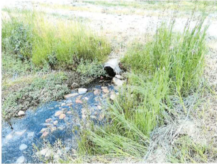
BOQUET CREEK INLET 18" OLD CROSSING
