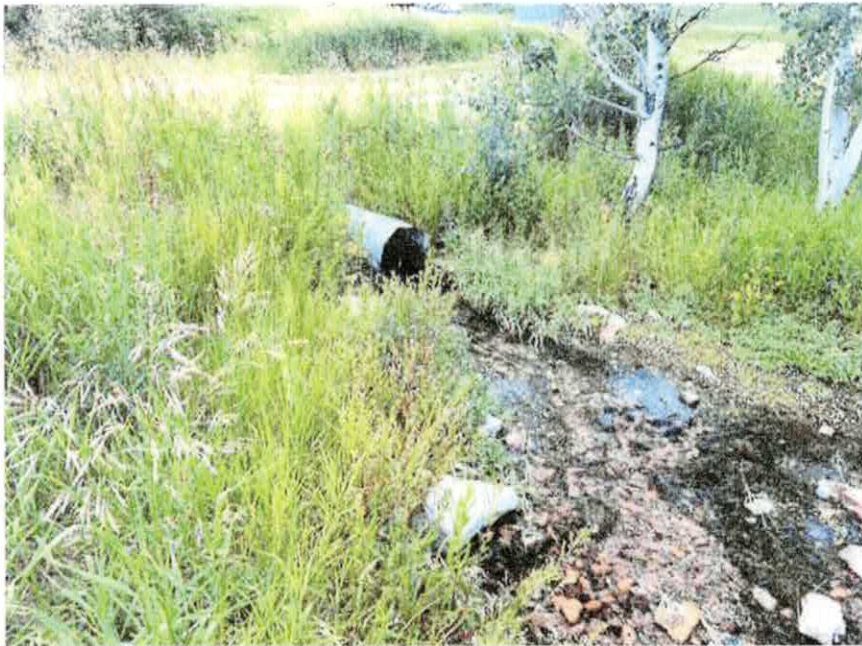
BOQUET CREEK OUTLET 18" OLD CROSSING
