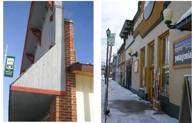
False fronts on Little Avenue (right) and on Main Street to be removed with future redevelopment. Historic restoration is encouraged where the original materials can be successfully rehabilitated or restored.
