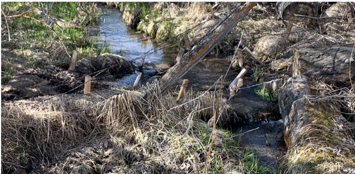
Figure 6. Photographic example of dilapidated straw wattles and the wooden stakes that used to hold them in place, at a location where surface waters exit the subject property within an altered spring creek stream channel, April 23, 2025.
