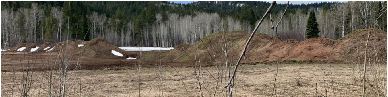
Figure 11. Photographic example of loose soil stockpiles and extensive area of vegetation removal and site disturbance that lack silt fence or other devices to prevent additional mobilization of fines from the subject property, April 23, 2025.
