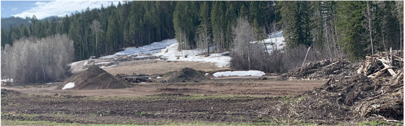
Figure 8. Photographic example of large expanse of disturbed ground and numerous stockpiles of loose soil that lack silt fence or other devices to prevent additional mobilization of fines from the subject property, April 23, 2025. The photograph also depicts some of the stockpiles of the woody vegetation that was removed from riparian and wetland areas.
